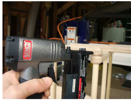
A pin nailer can be used to help hold the outer slats in place.
