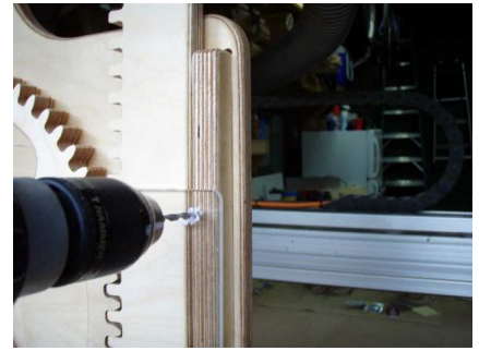
Pilot hole two holes into the Plexiglas over the rack support.
