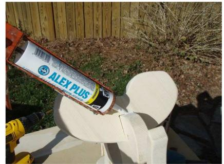
Run a small bead of caulk around the joint of the elephant ear and body parts. This will harden and give a nice look once the paint is applied.
