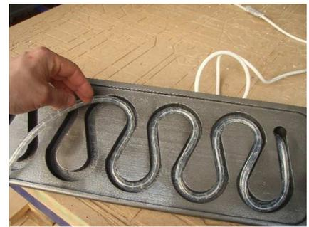
Start with one end and fish the rope through the channel. Make sure it isn't twisted up too much or the rope will have a tendency to pop out of the grooves.
