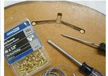
**fig. 5b** Install with Screws
