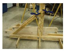
Glue and screw the diagonal pieces so they attach to the rear of the base and to the main arm assembly. Position the two arm pieces into the slot.
