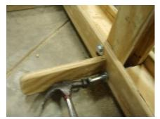
Strengthen this point with some bolt on hardware. 3/8" or 7/16" diameter will work fine, use whatever you have laying around the shop.
