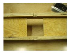
Make sure the space left in the middle of the base is wide enough to fit the main arm assembly of this project. It is a good idea to check this before the glue has had time to setup.
