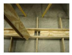
Set the main arm assembly onto the base. Wood screws or nails can be used to temporarily hold it in place.
